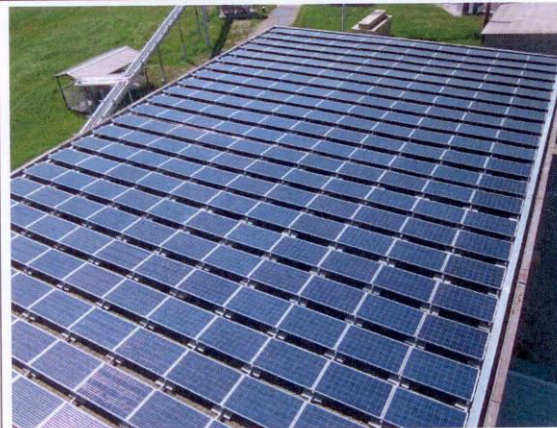
Picture 7: Top view roof 11
