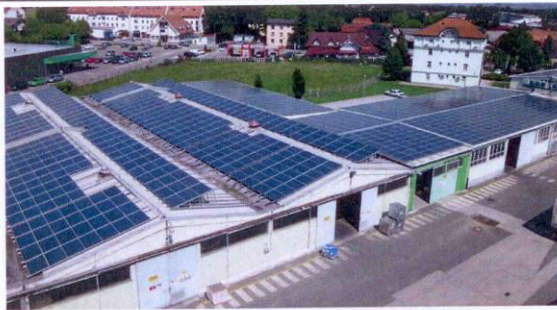
Picture 5: View from the right to roof 5, 5.1, 12.2 and 12.1
