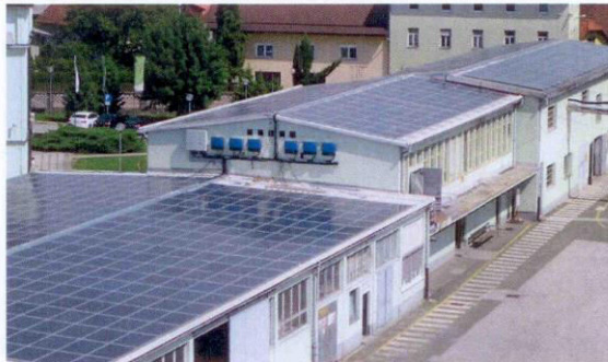
Picture 4: View from the right to roof 3, 4 and 5
