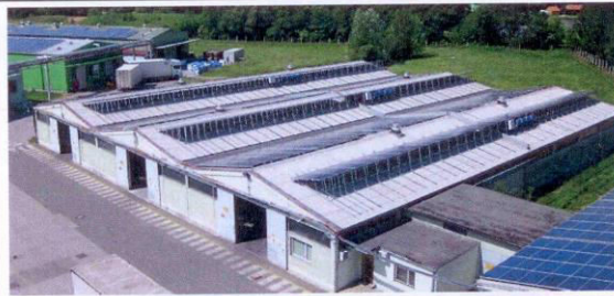
Picture 6: View from the right to roof 14.2, 14.1 and 14
