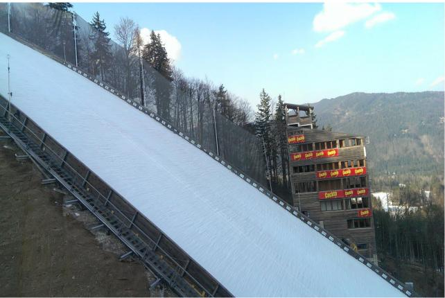
The flexible wind protection system can withstand wind gusts up to app.15 m/s If wind forecast is that there might be a constant wind of more than 12 m/s the system should be reffed and lifted again after the wind gets normal. The procedure of reffing or lifting can be effected in app. 4 minutes.
